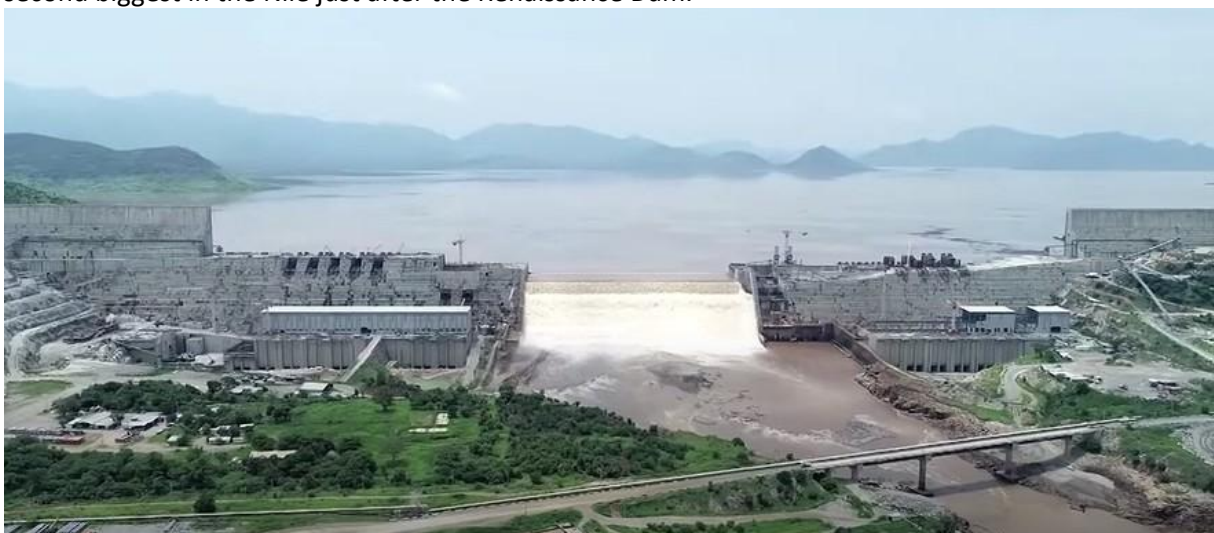
*Renaissance Dam in Ethiopia
